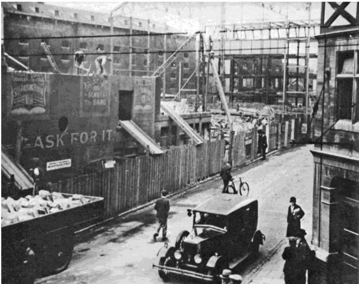
The New Inn during the demolition of the Post Office on the opposite corner. The construction of the Forum can be made out in the background.
